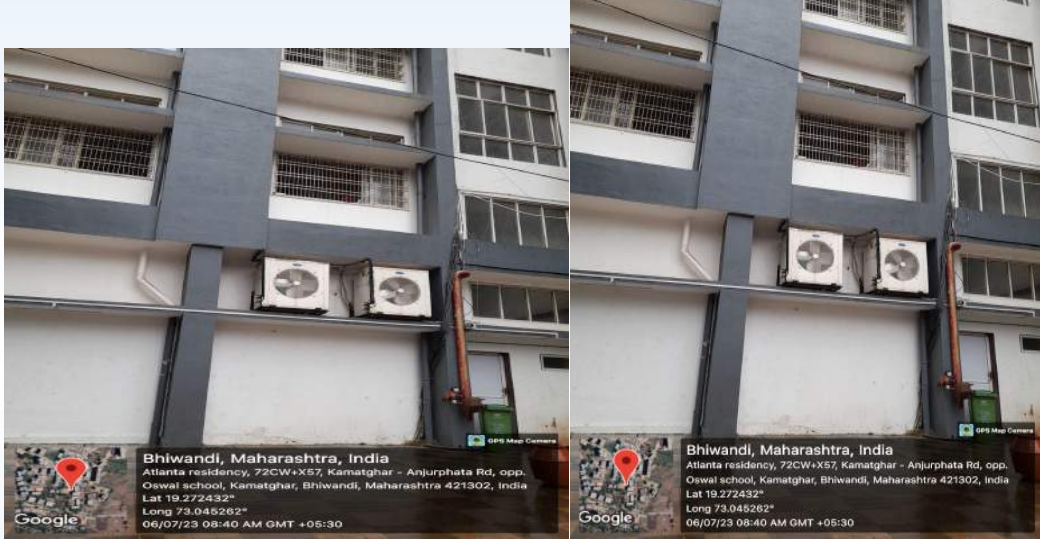
RAIN WATER CONSERVATION FROM TERRACE TO GROUND (SEQUENCE IN PICS FROM LEFT TO RIGHT)
